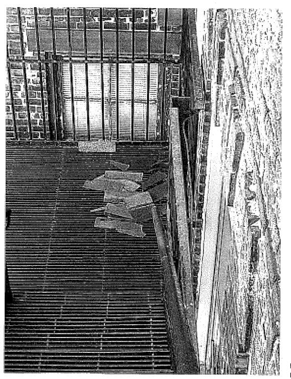
Fire escape: Roof shingles falling off roof.
