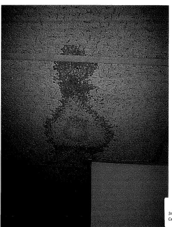
3rd floor Hallway: Ceiling tile, water damage and mold.
