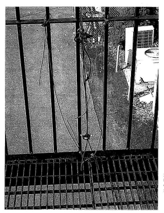
2<sup>nd</sup> floor Fire Escape: Landing fell-repaired by welding. Cables attached for a little extra Safety.
